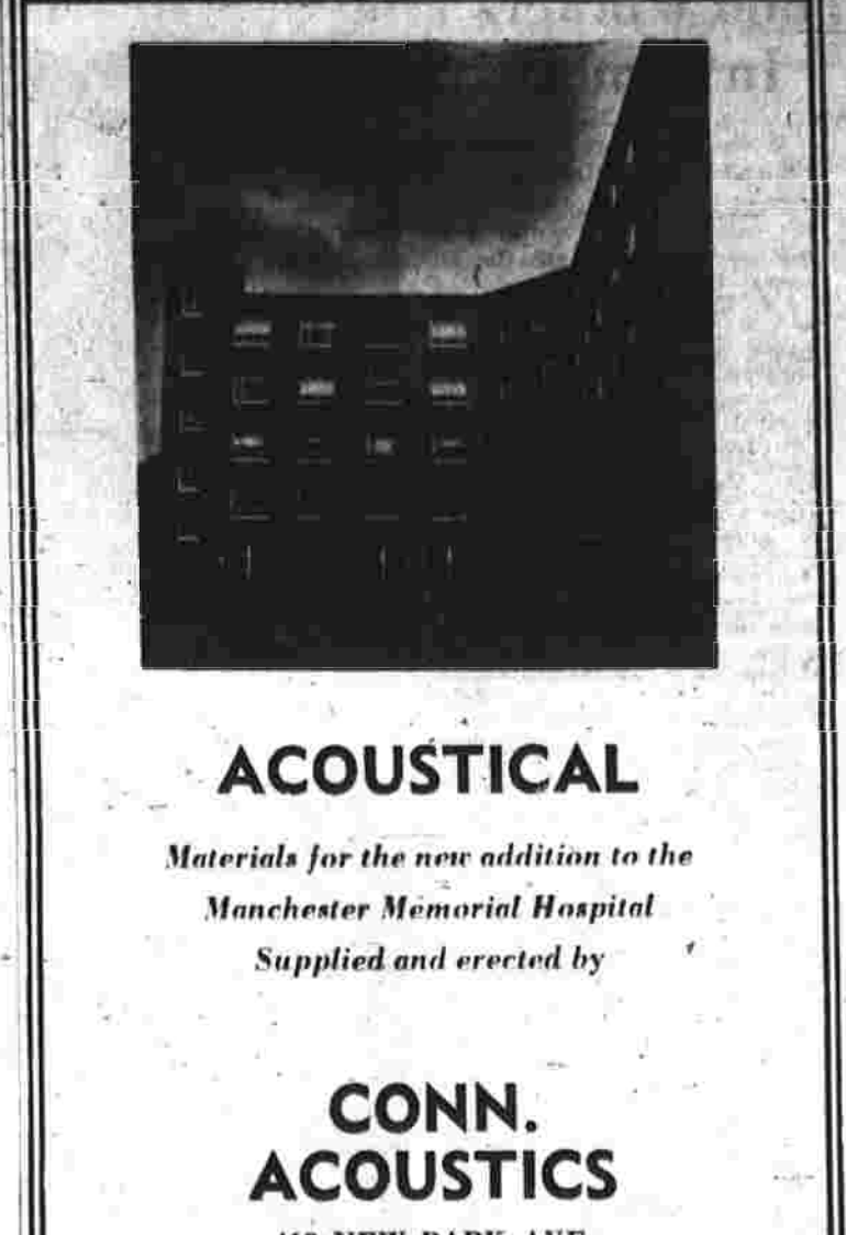
Materials for the new addition to the Manchester Memorial Hospital. Supplied and erected by
